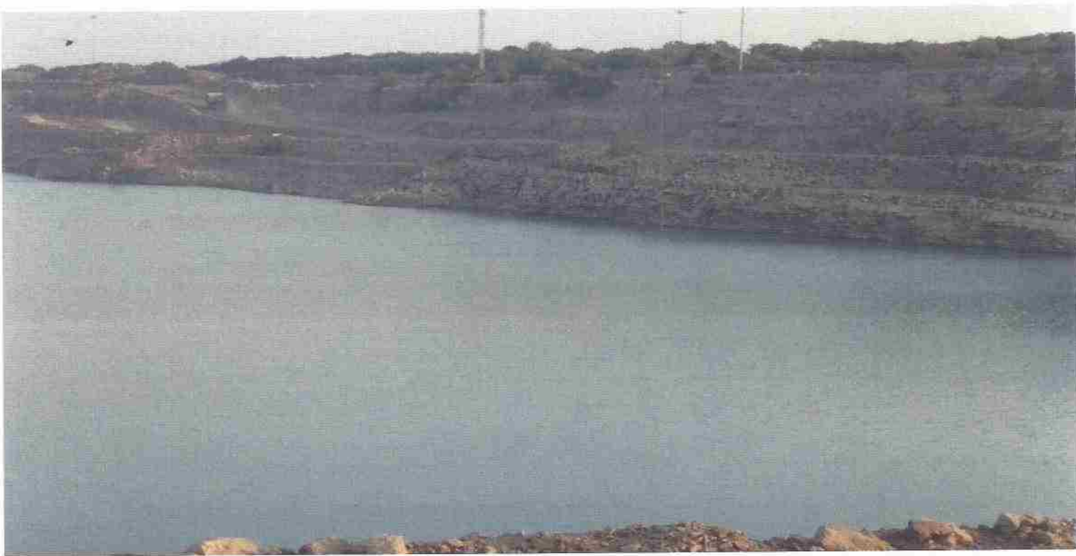
CONSERVATION MEASURES TO AUGMENT GROUND WATER AND COLLECTION IN MINE PIT
